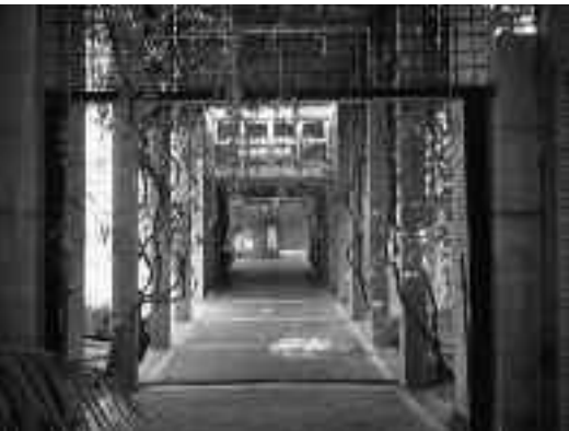
Ecole ATAM, Seville - SAMA architectes
